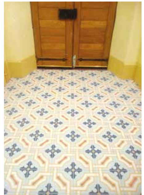
The new tiles in St. Maeldoid's Church.
