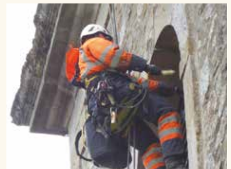
A rope access specialist cleaning the louvres in the Cathedral.
