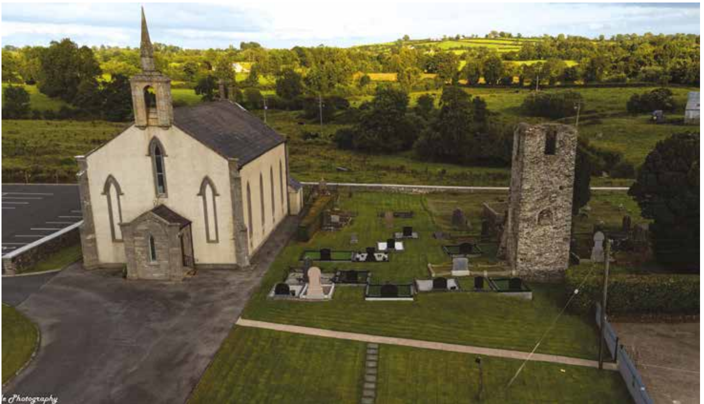
An aerial photo of St. Colman's Church, Clontibret.
