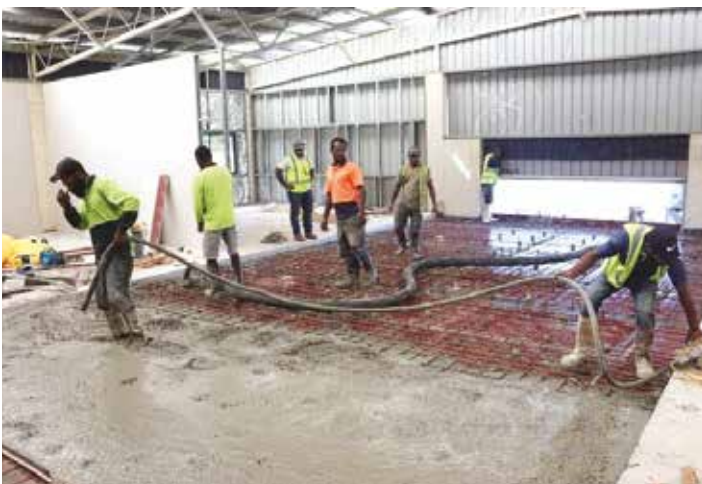
Renovation of the YHAM headquarters underway.
