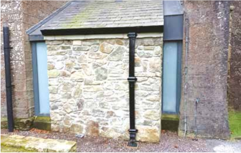
The exterior of the toilet extension.
