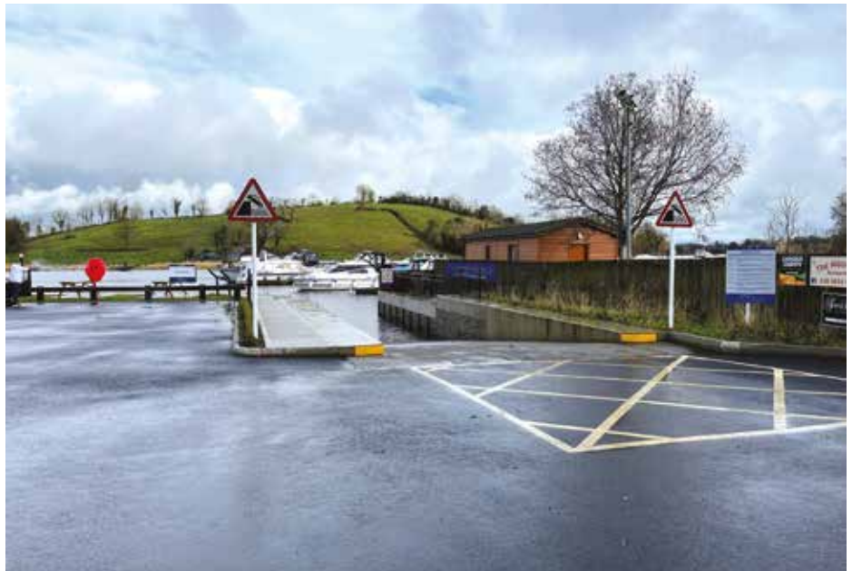
The warning signs at the new slipway.
