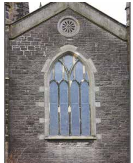
The restored east window.
