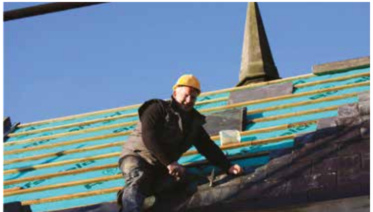
Patrick Gilheaney on the Chapter Room roof. Patrick, who is a specialist in slating, fitted all the slates on the cathedral roofs.
