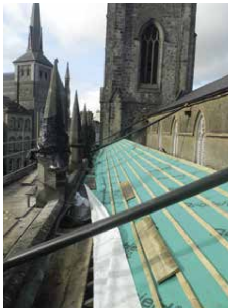
The newly felted and lathed south lower roof.
