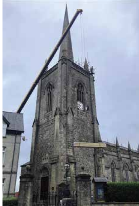
Scaffolding being removed from the tower.
