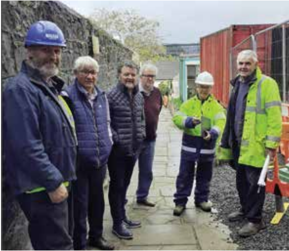
A post inspection meeting taking place with (from left): Mr David Hall, site manager; Mr George Irvine, glebewarden; Mr Marius Blake, quantity surveyor; Mr John Muldoon, quantity surveyor; Mr Chris McCollum, conservation specialist; and Mr Harold Graham, contractor.
