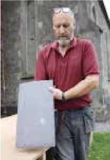
Mr David Hall, Harold Graham's site manager, showing a new slate with the copper nails and clip in position. The specialist slaters have made a good start on fixing the slates on the south facing slope of the cathedral's high roof.
