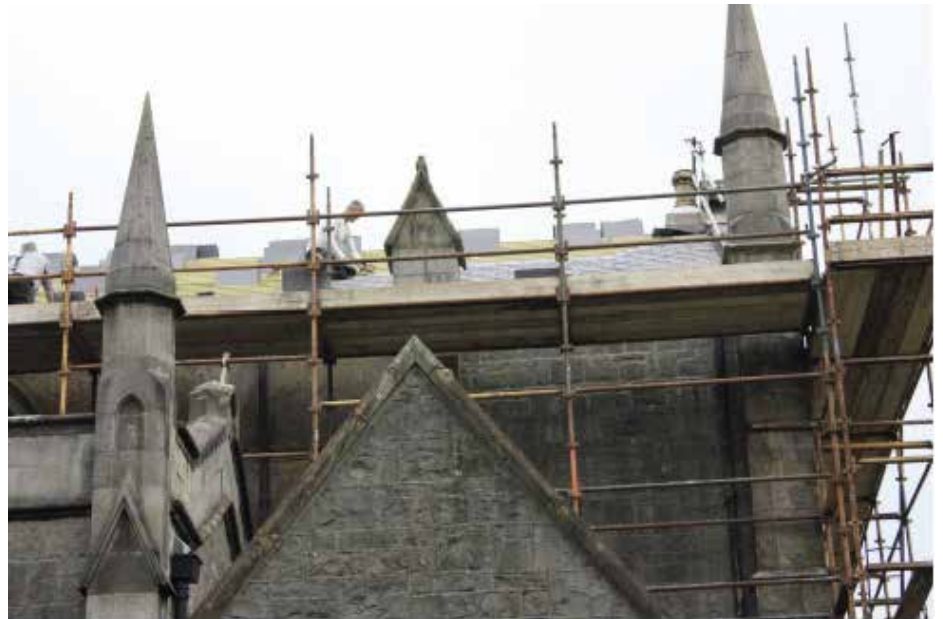
Mr David Hall, Harold Graham's site manager, showing a new slate with the copper nails and clip in position. The specialist slaters have made a good start on fixing the slates on the south facing slope of the cathedral's high roof.
