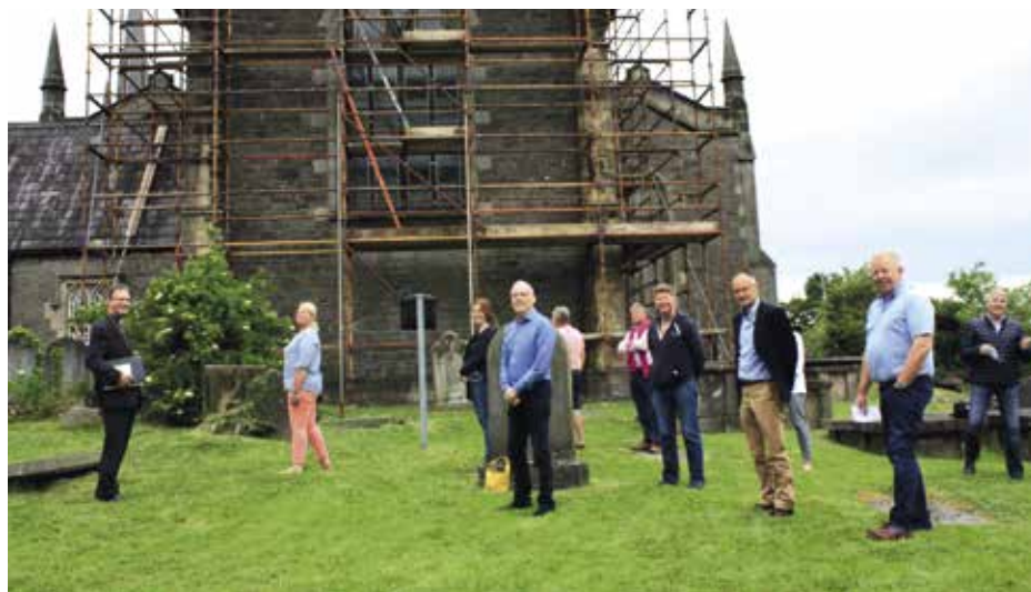
The Dean and parish representatives view the restoration work in progress.
