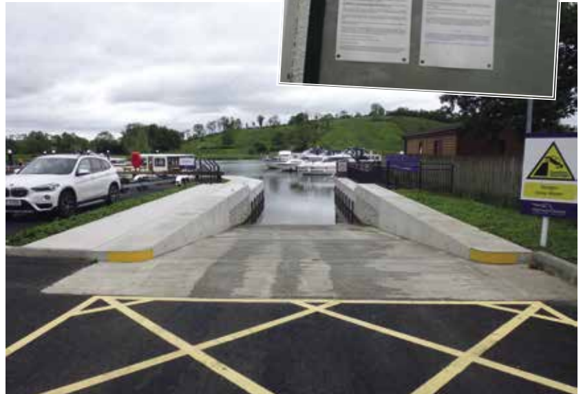
The new Slipway at Bellanaleck Quay.
