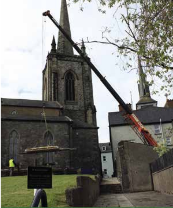
Heavy lifting machinery bringing scaffolding to the rear of the Cathedral.
