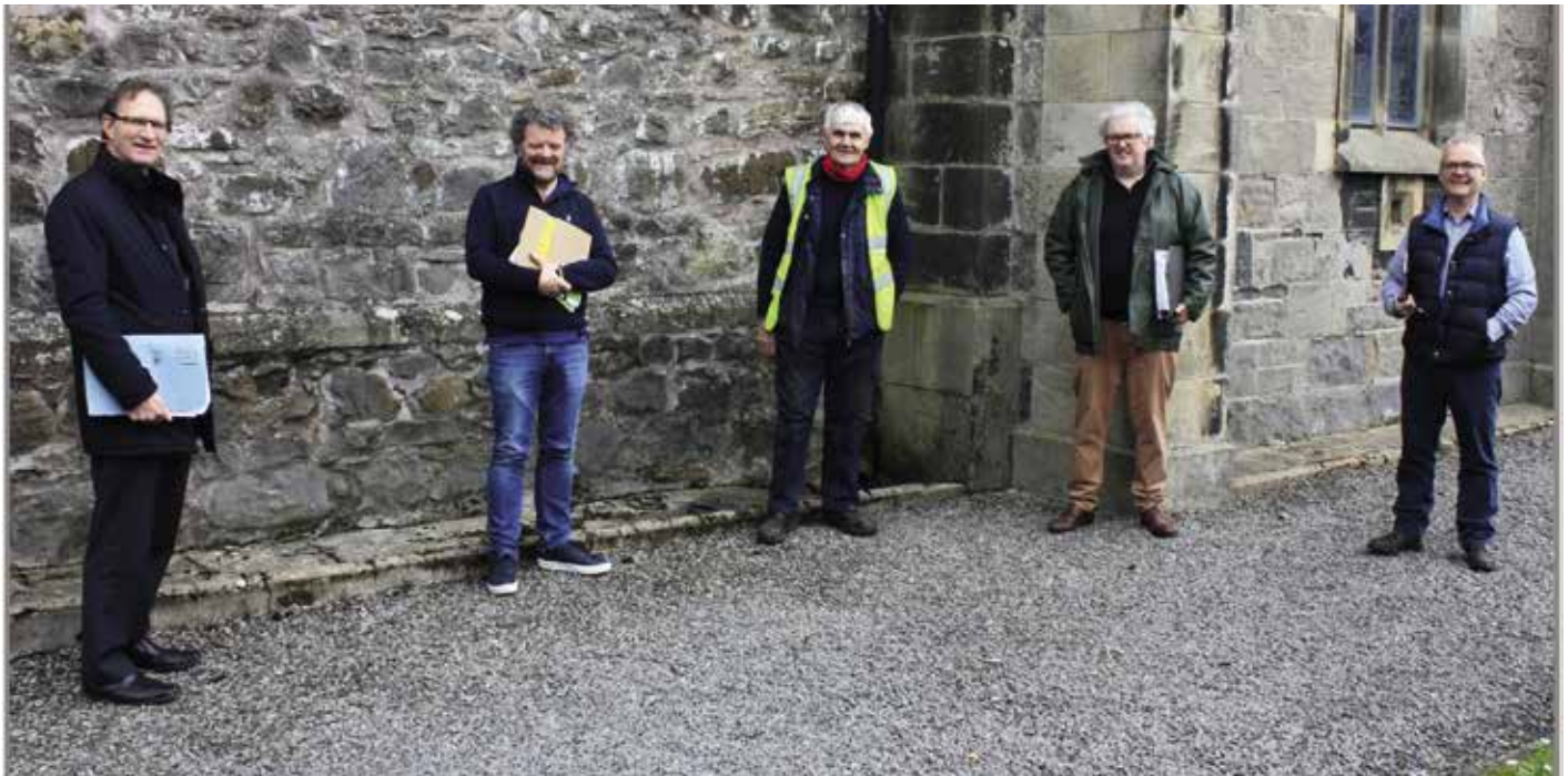
Discussing arrangements for the cathedral restoration work. With the Dean are from left: Mr Marius Blake; Mr Harold Graham, main contractor; Mr J Muldoon and Mr Chris McCollum, historic buildings restoration specialist, who will supervise the work. Messrs Blake and Muldoon are quantity surveyors involved in the project.
