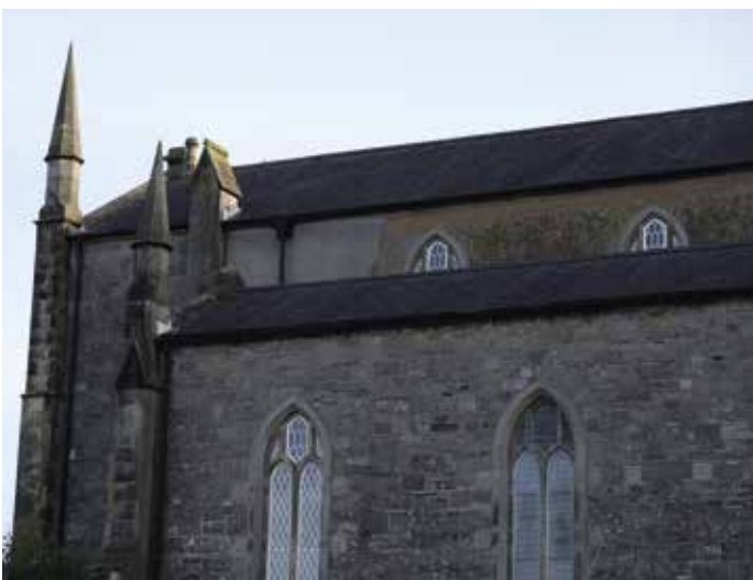
The high roof sections of St. Macartin's Cathedral.
