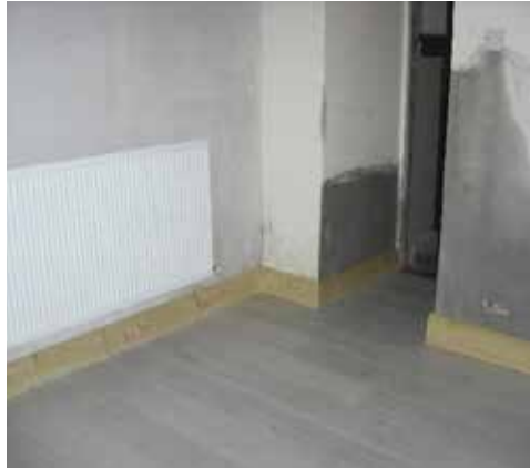
The Vestry Room with new radiators, replastering and new floor covering.
