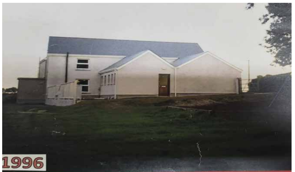
The Billis School was renovated in 1996.
