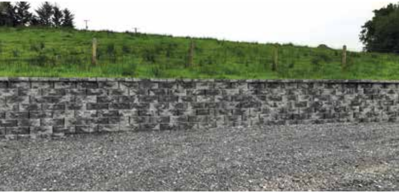
The newly built boundary wall of Mullaghduin Car Park.
