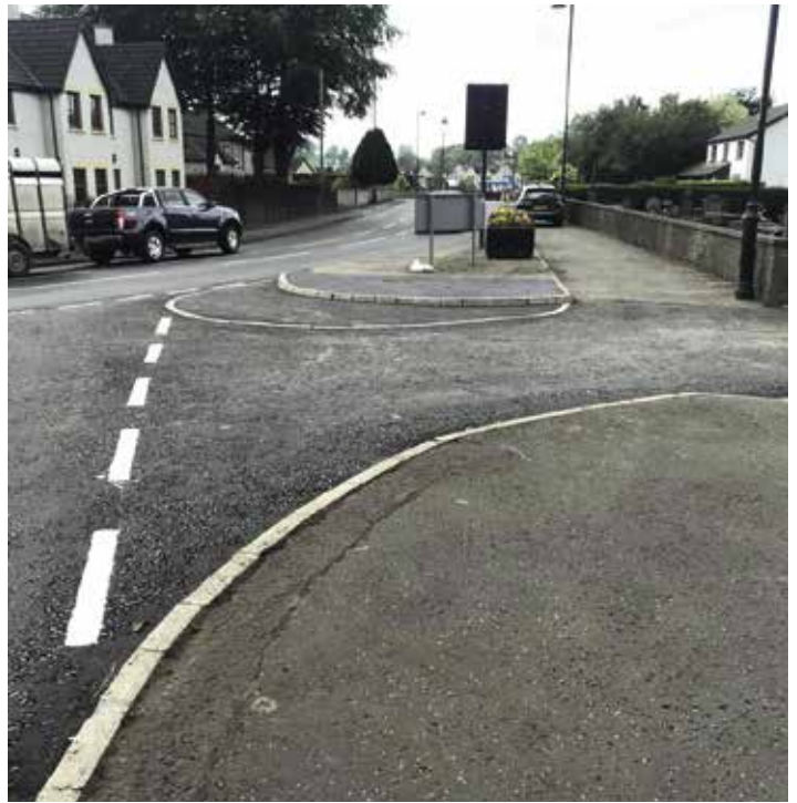
Construction of left turn into Cleenish Parish car park.
