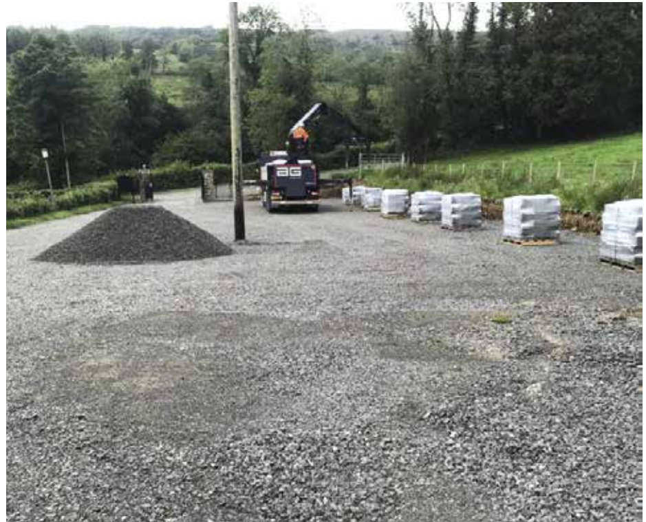
Constructing the new car park at Mullaghduin.
