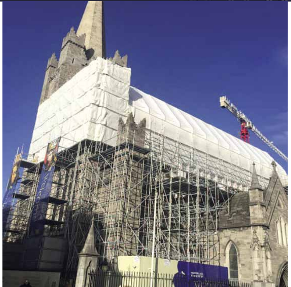
St. Patrick's Cathedral surrounded by scaffolding while roof repairs take place.
