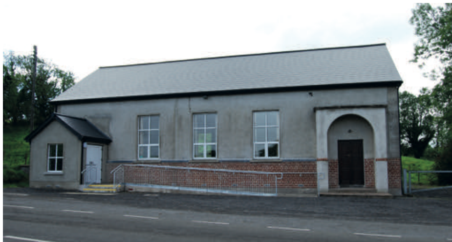
Derryvullen South Parish Hall, Tamlaght.
