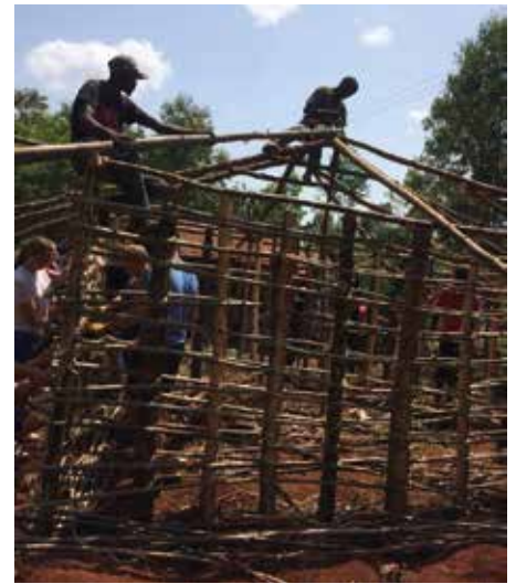
The frame of the house goes up.
