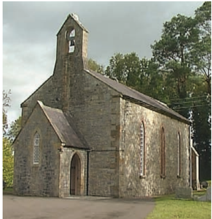
St. Michael's Parish Church, Derrybrusk
