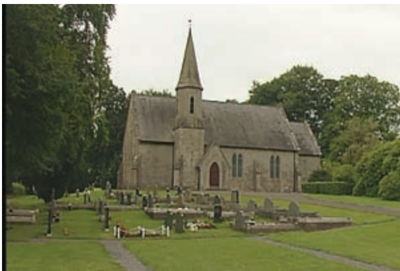
St.Tighernach's Church, Derryvullen South, Tamlaght.
