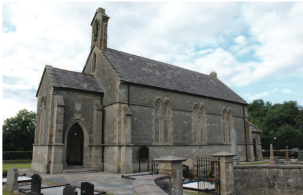
The new roof on Drummully
