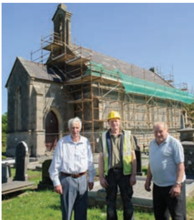
George, Robert and William with work at Drummully nearing completion
