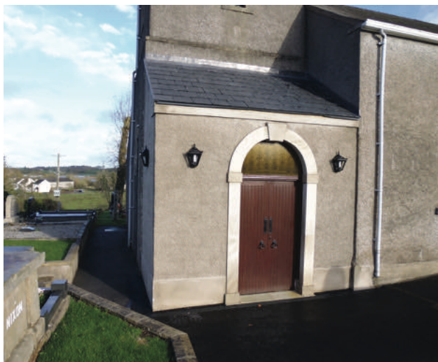
Extension to Cleenish Church porch
