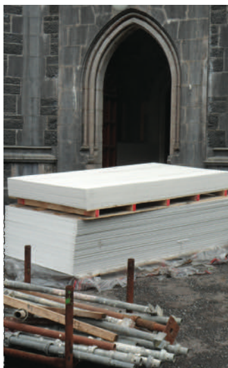
New ceiling ready to go in
