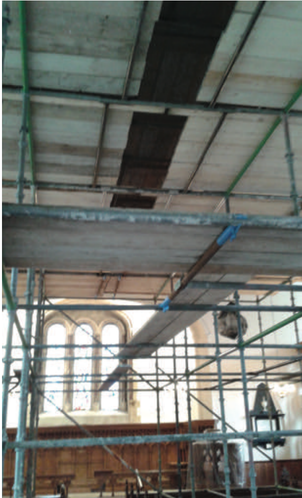
Scaffolding in the Church
