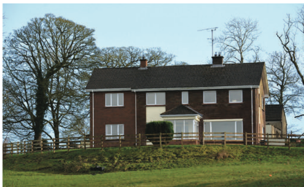
Newly re-furbished rectory
