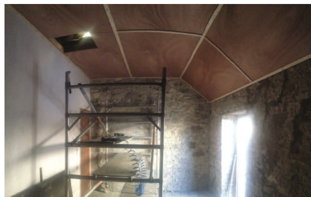
Early work in progress
