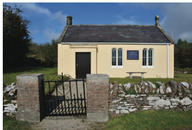
Coolbuck Church pictured after the capstones had been stolen
